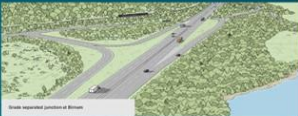
All dual carriageway includes a 150m long underpass with Station Road connection to the Dunkeld & Birnam Railway Station
