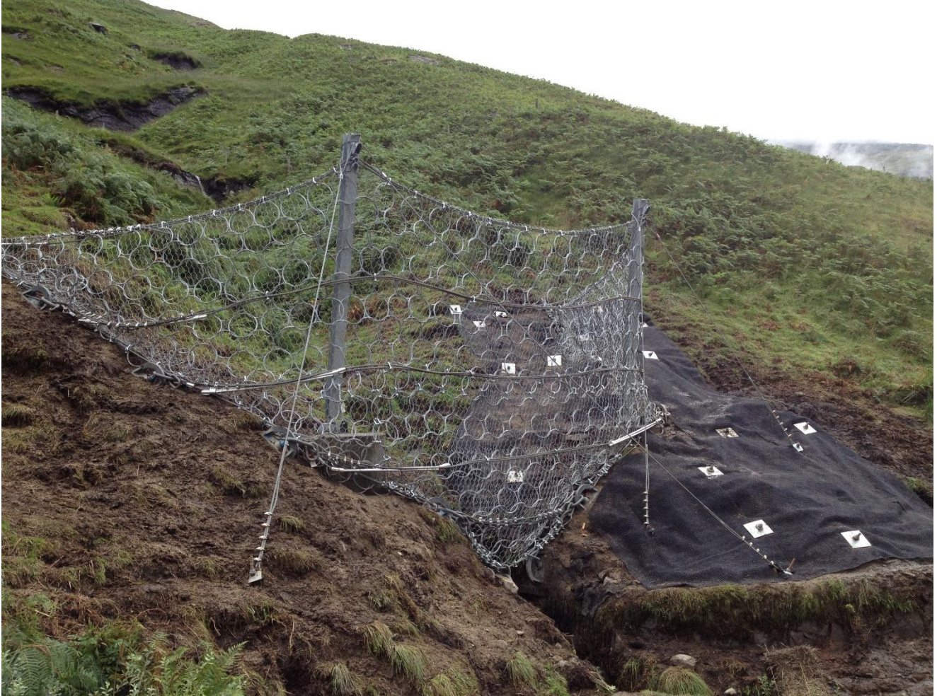
Figure 2-5 – Typical example of an in-channel barrier on the Beinn Luibhean hillside
