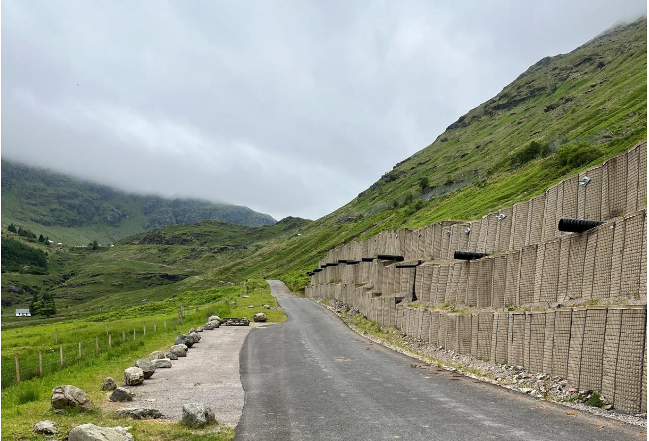
Figure 2-15 – HESCO Barrier, looking north towards the Rest and Be Thankful Viewpoint Car Park with Beinn an Lochain (left) and Beinn Luibhean (right) in the background
