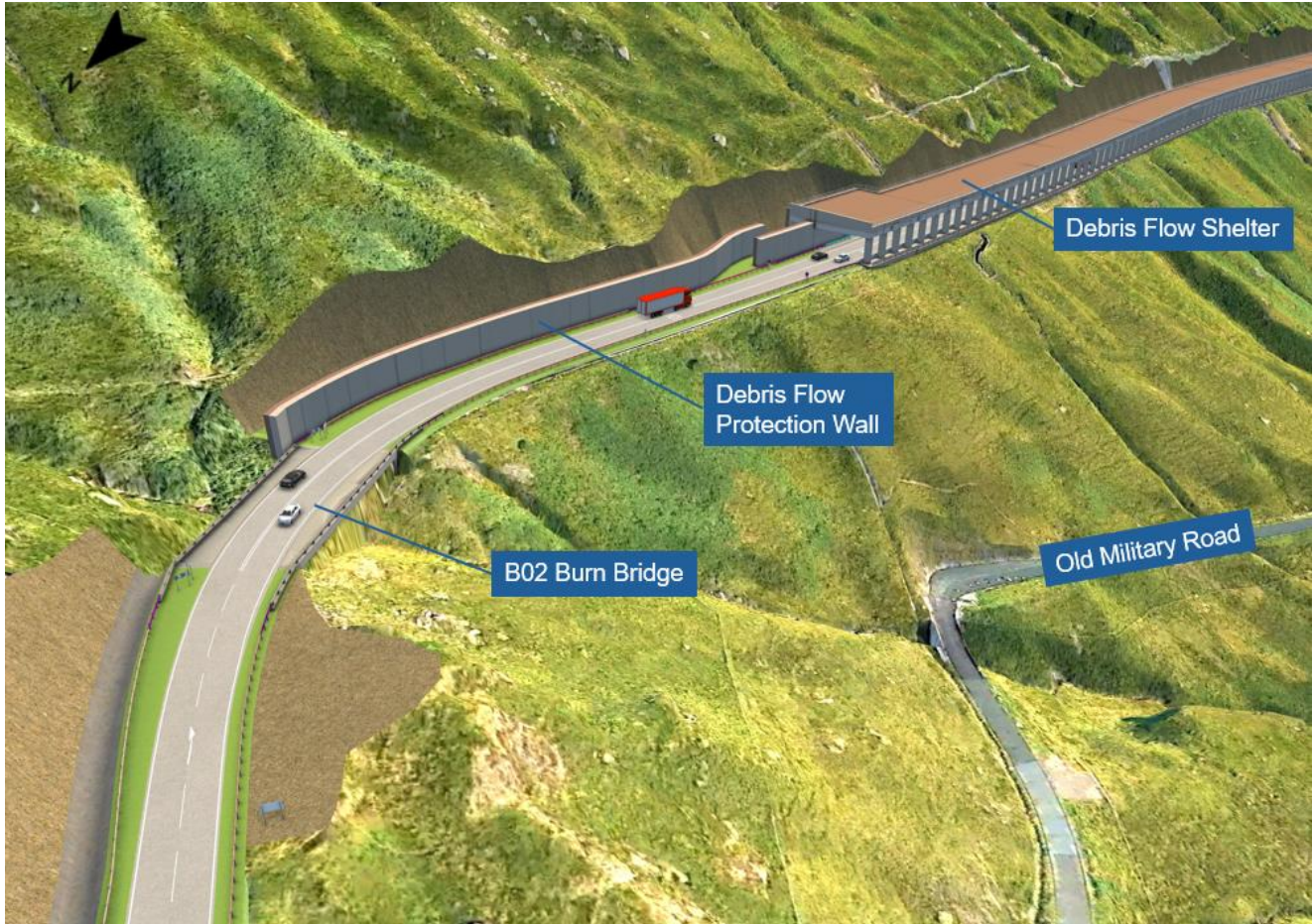
Figure 3-8 – Computer generated image of the DFW at the northern end of the Proposed Scheme
