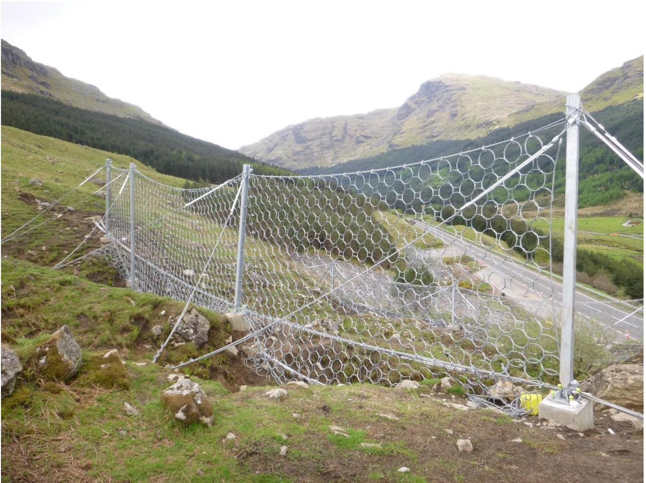
Figure 2-4 – Typical example of a shallow landslide barrier on the Beinn Luibhean hillside
