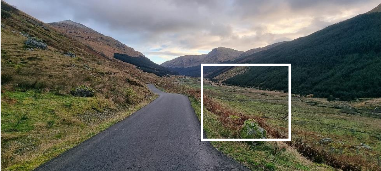
Figure 2-11 – OMR Retaining Wall 1, looking south with The Cobbler (left) and The Brack (right) in the background
