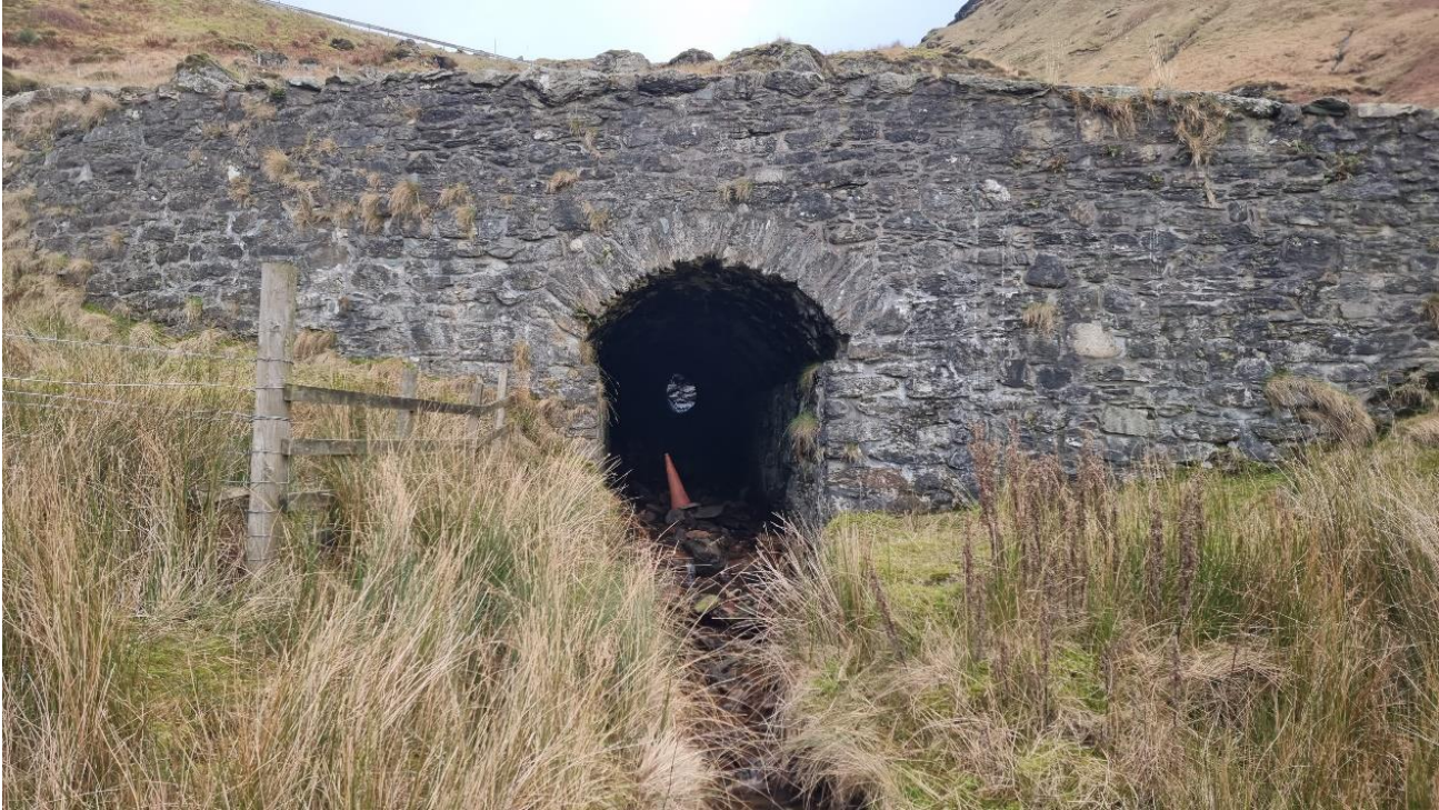
Figure 2-10 – OMR Bridge C, Western Elevation
