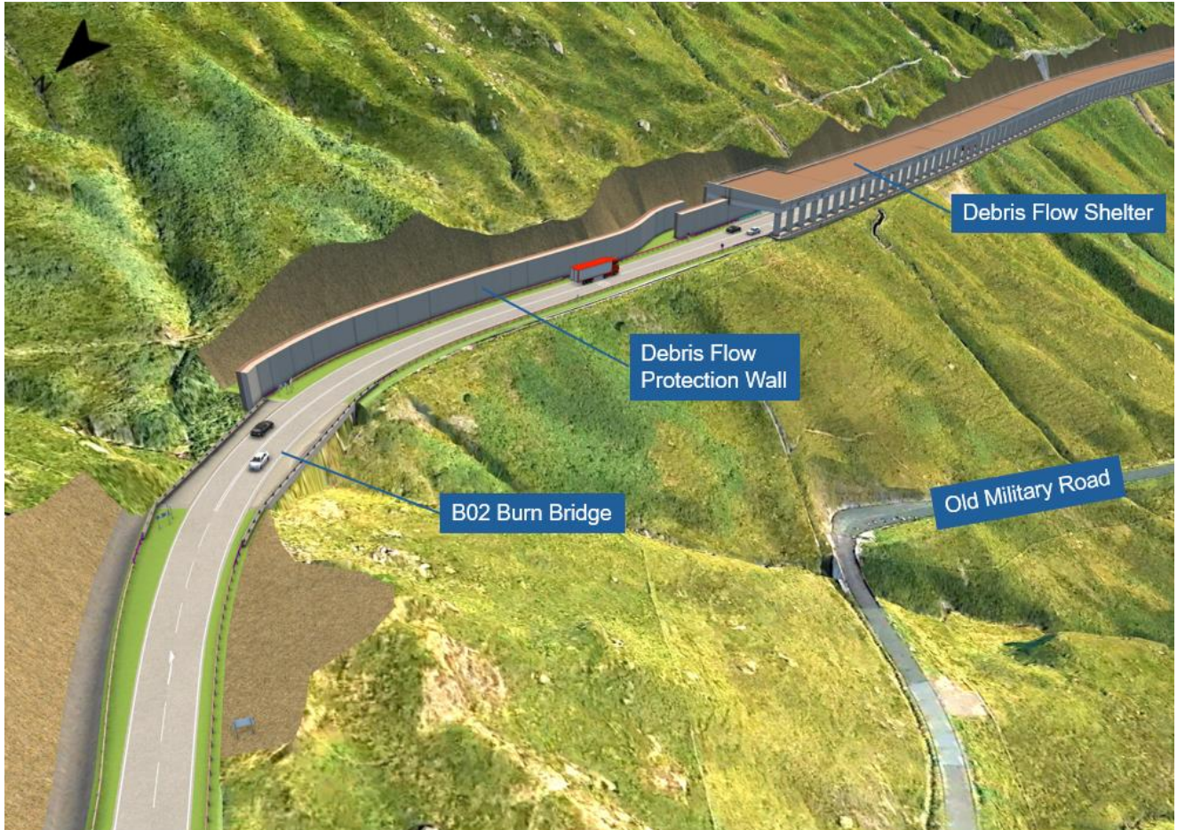
Figure 4-5 – Computer generated image of the DFW at the northern end of the Proposed Scheme
