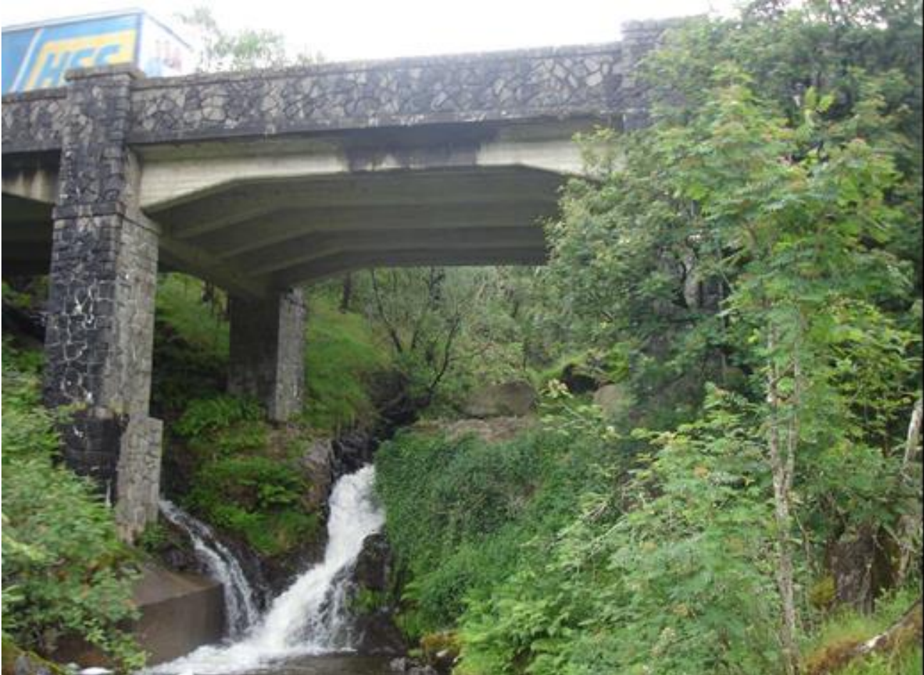
Figure 2-7 – Western elevation of The Cobbler Bridge, looking east up Croe Water
