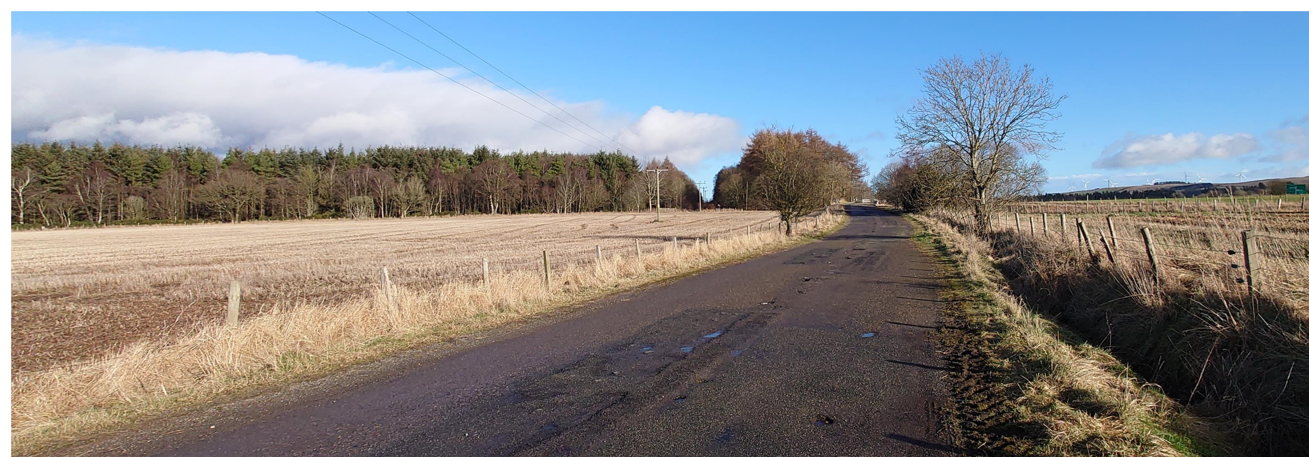
Existing U91K and surrounding landscape including Denlethen Woods at Oatyhill Rail Bridge
