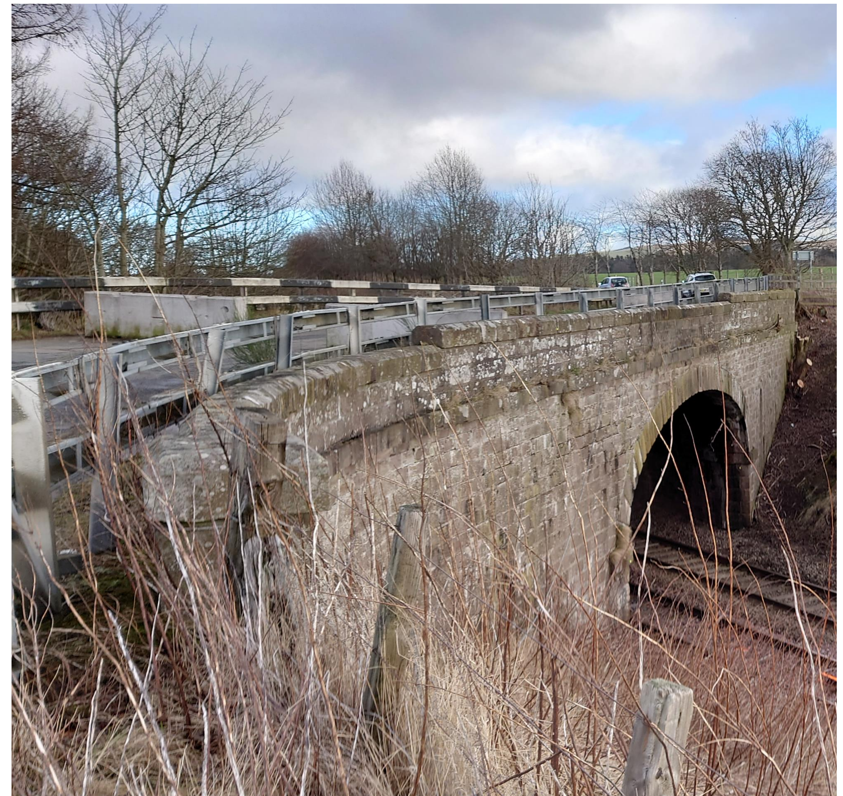
Oatyhill Rail Bridge looking northwest
