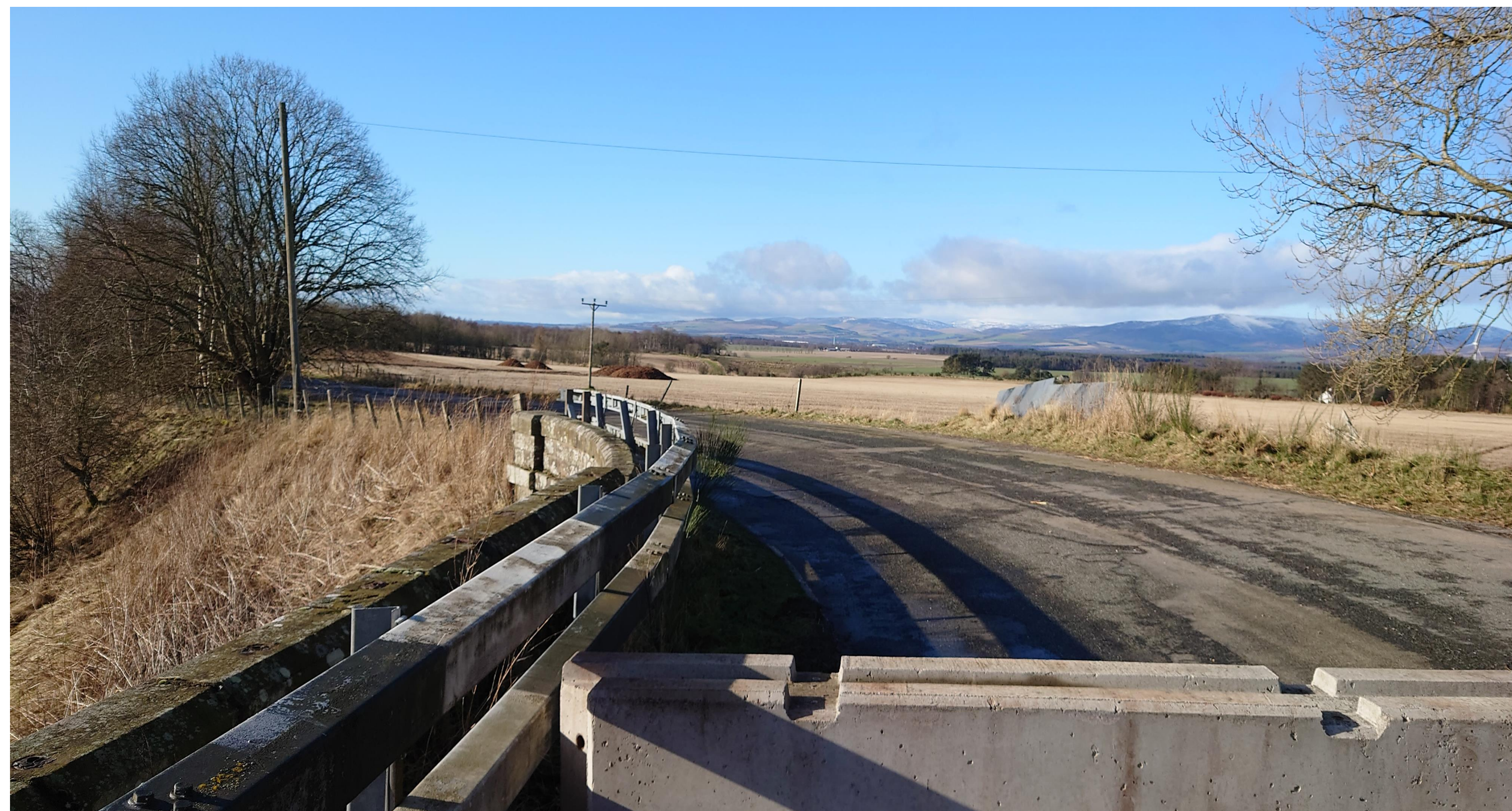
Existing U91k from Oatyhill Railway Bridge and surrounding landscape looking south by Denlethen Woods
