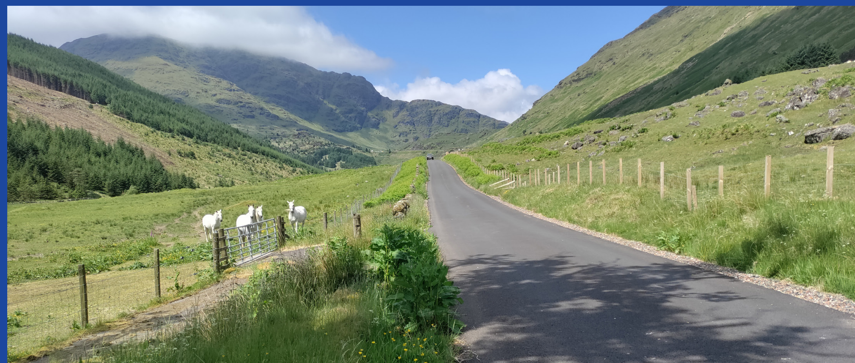
View along the OMR within Glen Croe looking northwest
