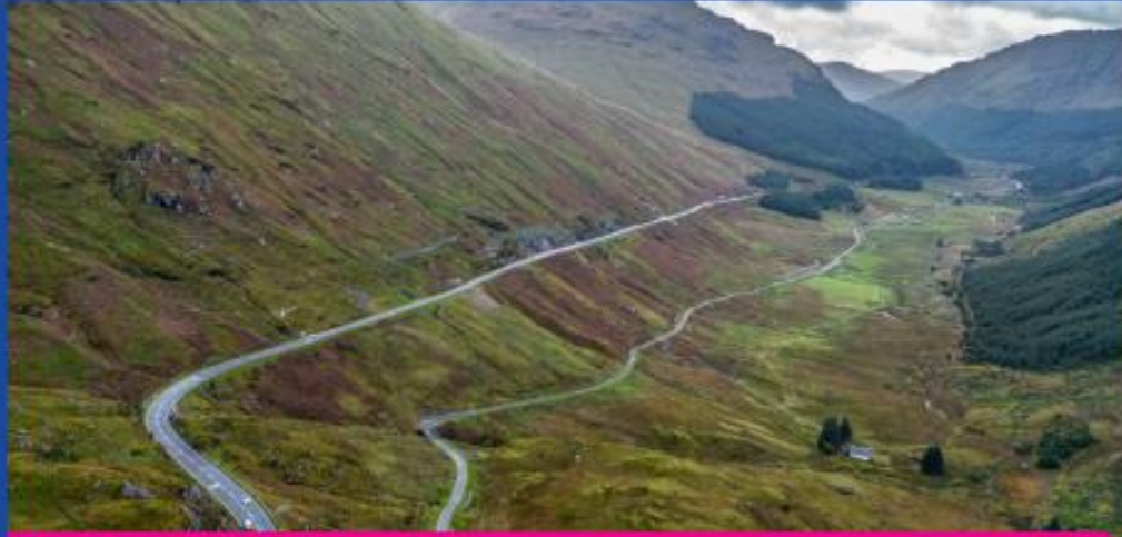
Aerial image of A83 and Old Military Road looking south east
