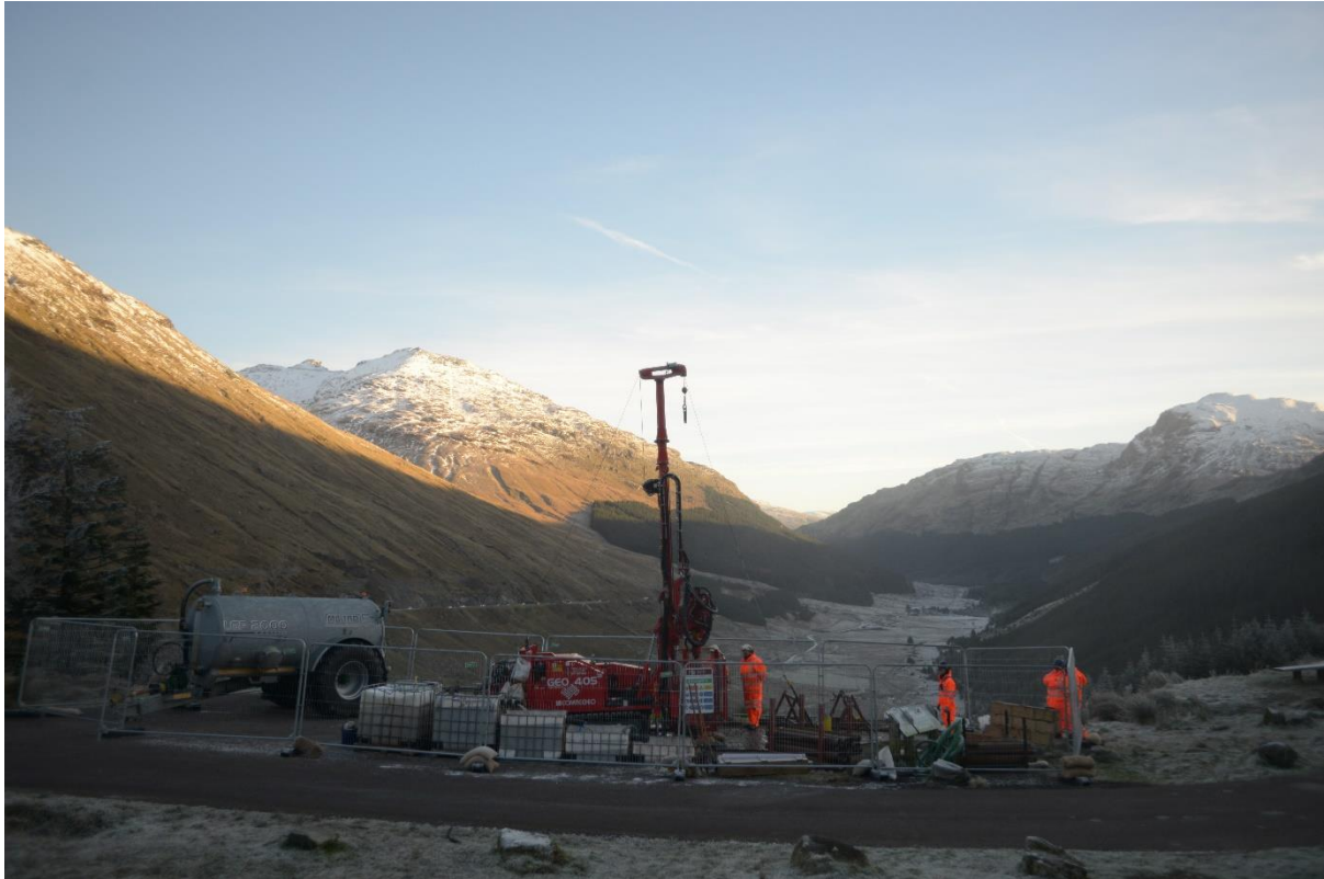
Figure 2 Ground Investigation work being undertaken at A83 Rest and Be Thankful
