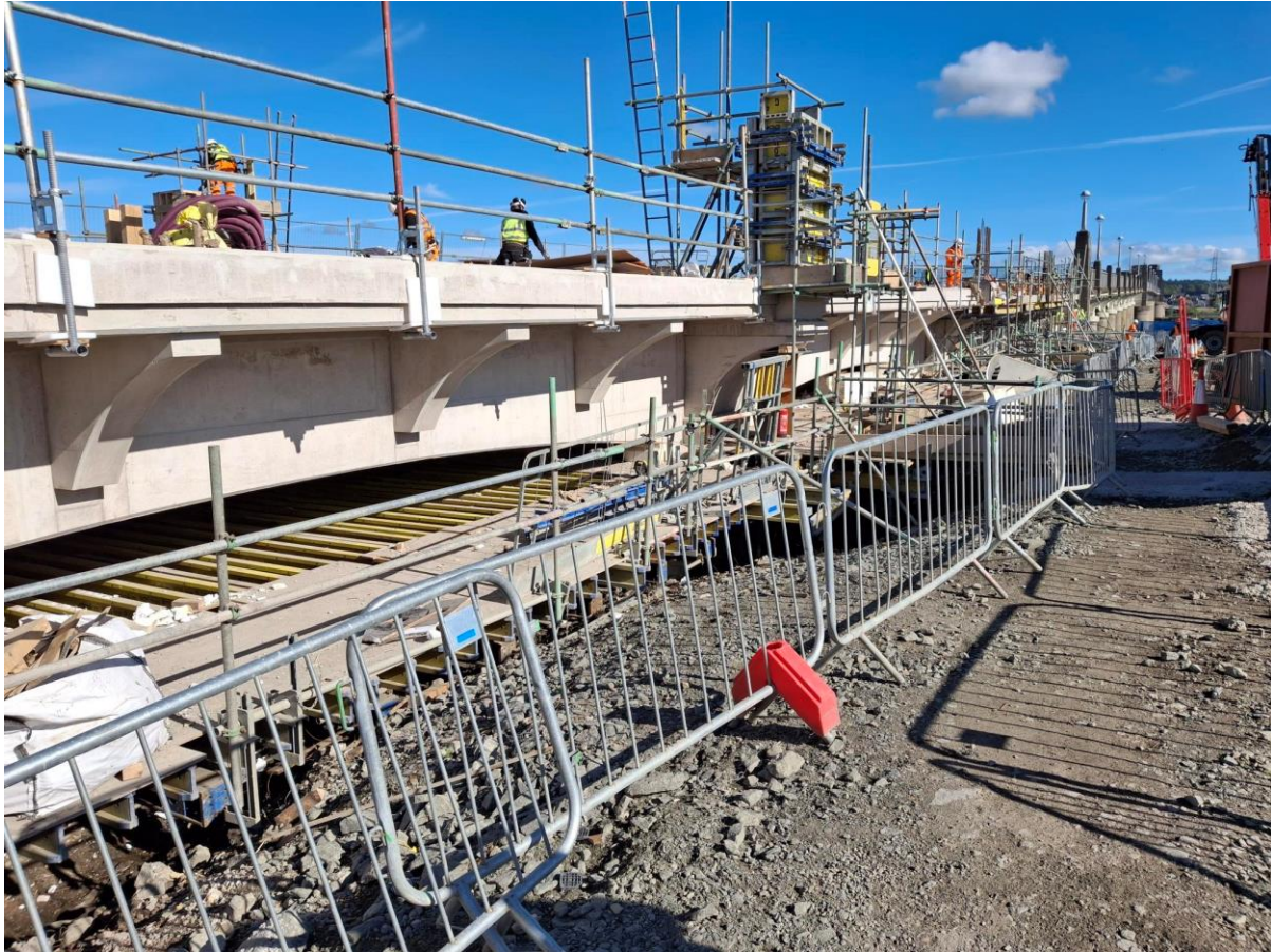
Figure 7 A985 Kincardine Bridge Southern Piled Viaduct replacement
