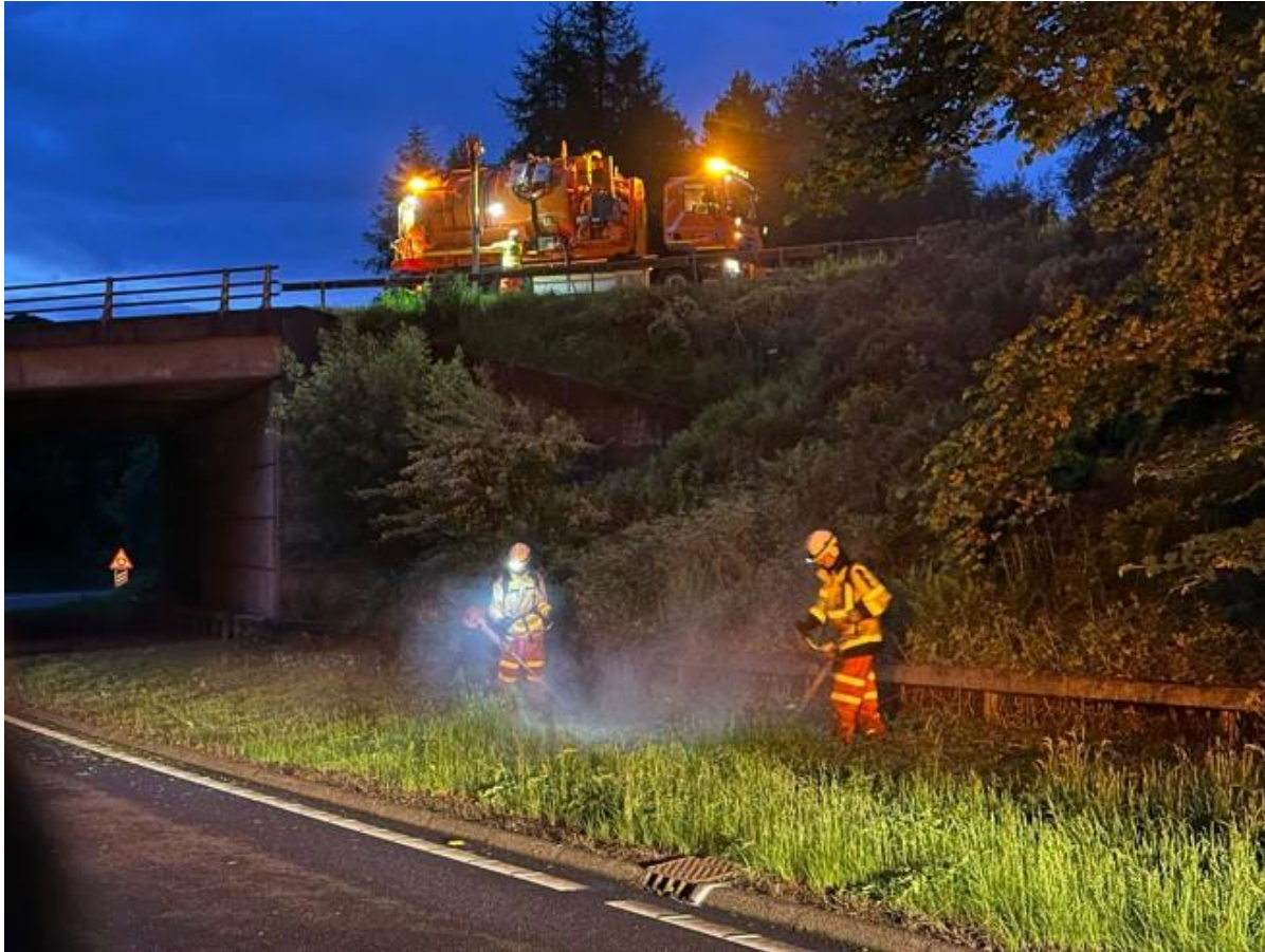
Figure 6 Operatives undertaking routine maintenance on the Trunk Road Network
