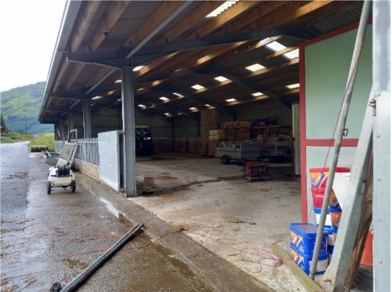
Photograph 15: Target Note ID – PM13, large agricultural building with an open side.
