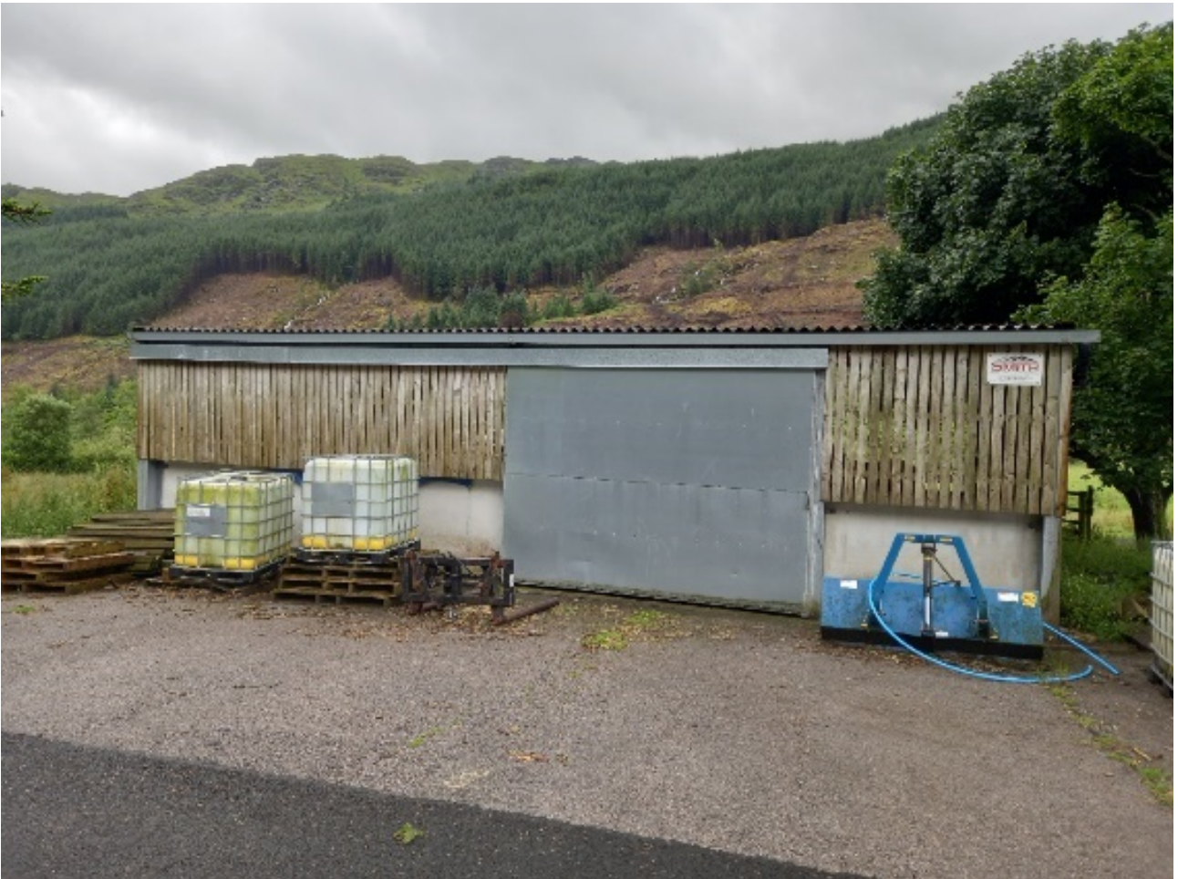
Photograph 16: Target Note ID – PM14, a stable building providing a suitable denning opportunity for pine marten.
