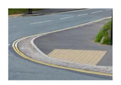
Dropped kerbs are the edge stones between a pavement and the road, that are lowered to make it easier for pushchairs and wheelchairs to cross over.
