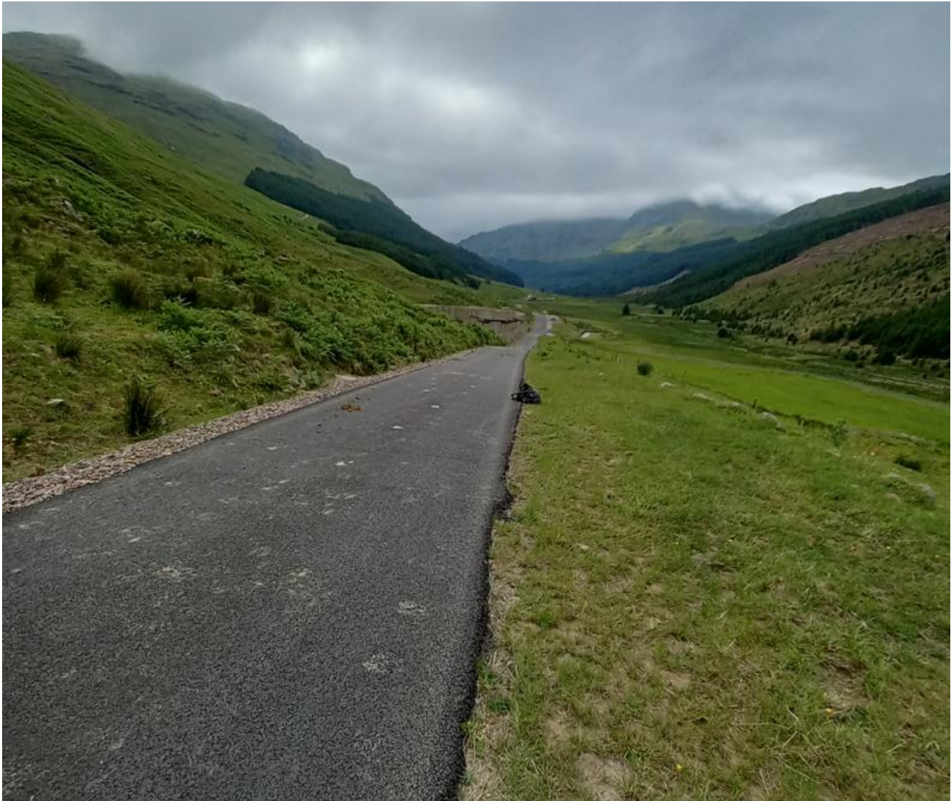
Figure 2 – A view along the Old Military Road within Glen Croe
