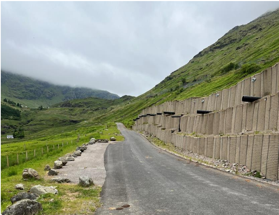
Figure 2-5 – Existing HESCO Barrier looking north-east along the OMR
