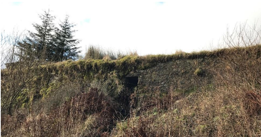
Figure 2-10 – OMR Retaining Wall 3, looking north
