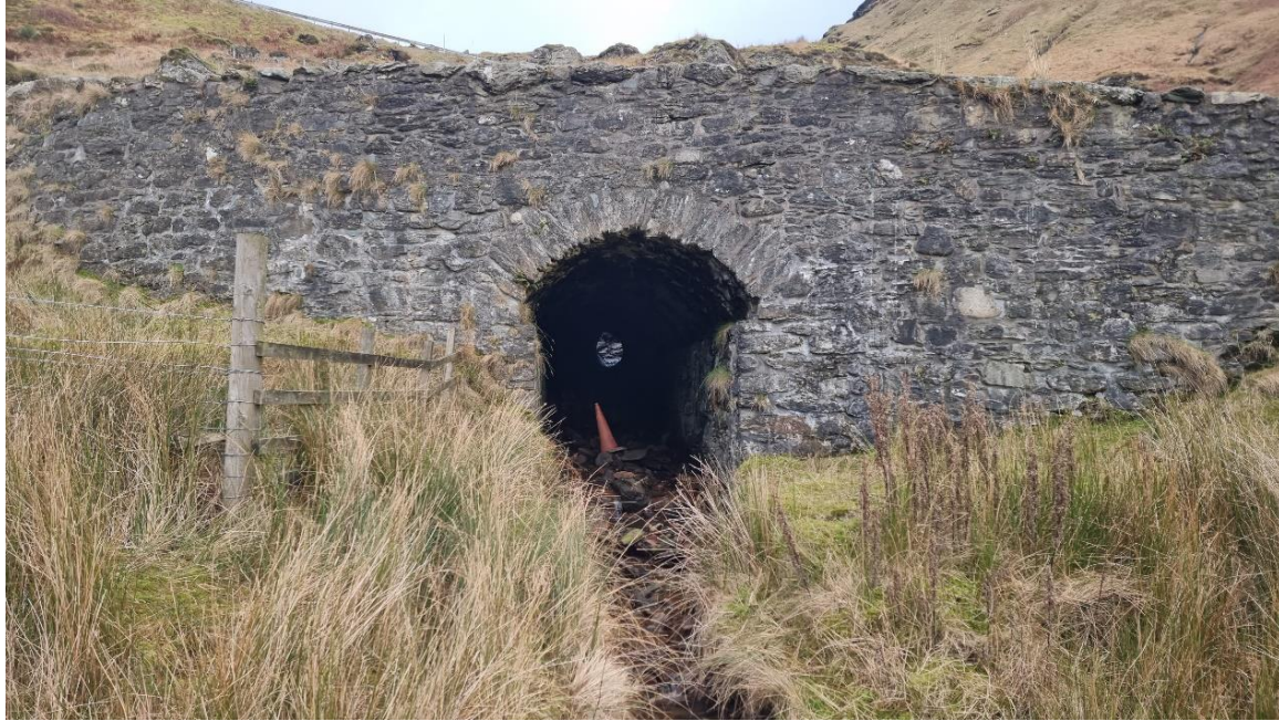
Figure 2-4 – OMR Bridge C, Western Elevation
