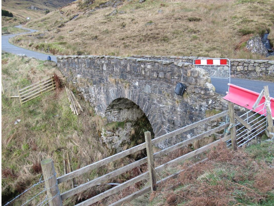
Figure 2-3 – OMR Bridge B, South-Western Elevation
