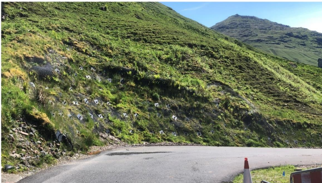
Figure 2-1 - Existing soil nailed slope on the OMR, looking east
