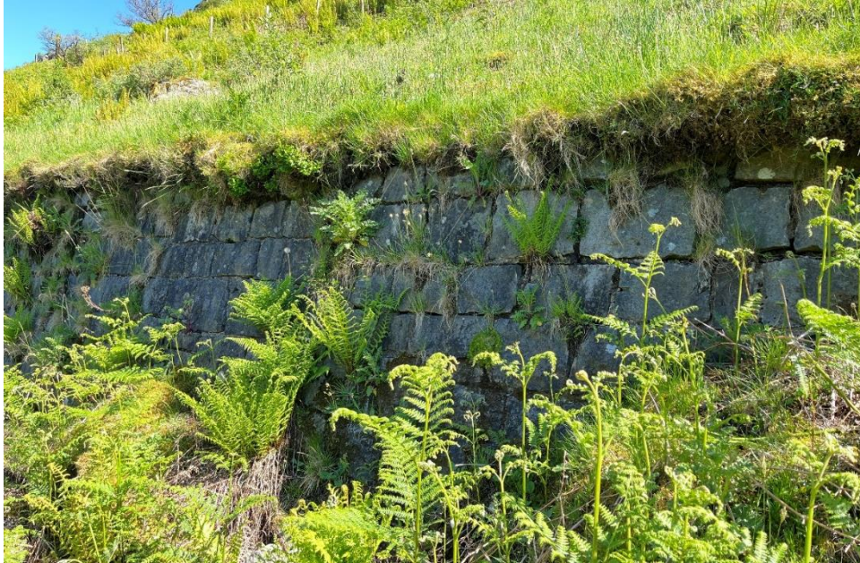
Figure 2-11 - Retaining Wall 4, looking north
