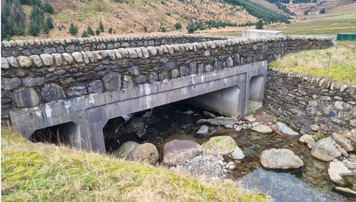
Figure 2-2 – OMR Bridge A, looking west down the Croe Water
