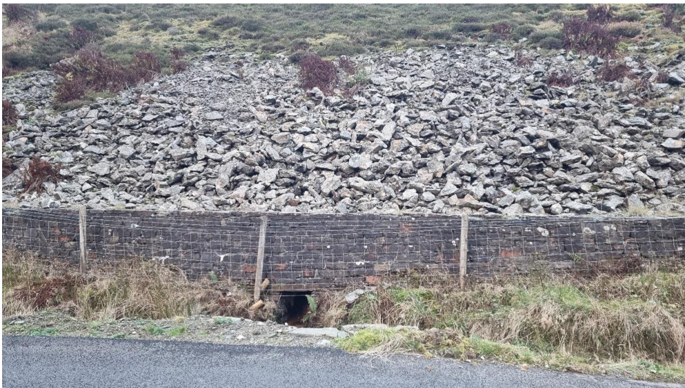
Figure 2-9 – OMR Retaining Wall 2, looking east
