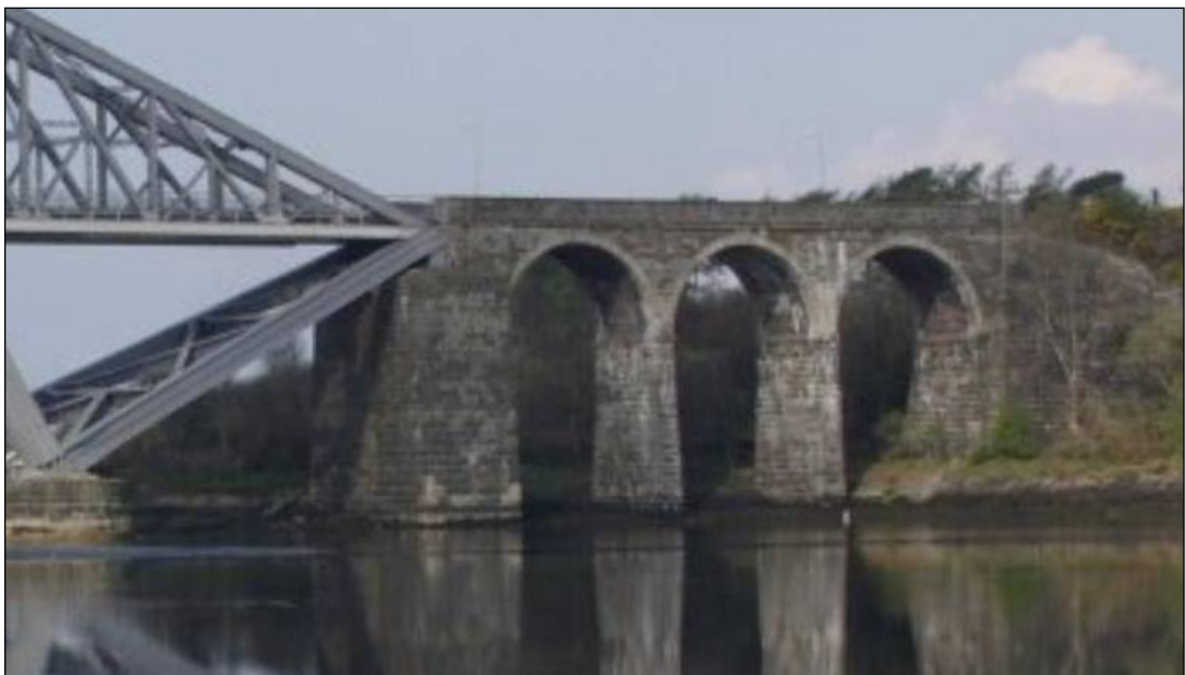
Figure 4.15.25.A – A828 11 Connel North Approach
