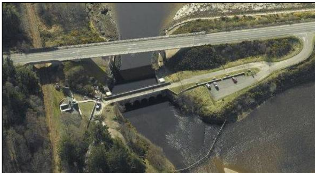
Figure 4.15.127.A – A9 1600 Mound Sluices
