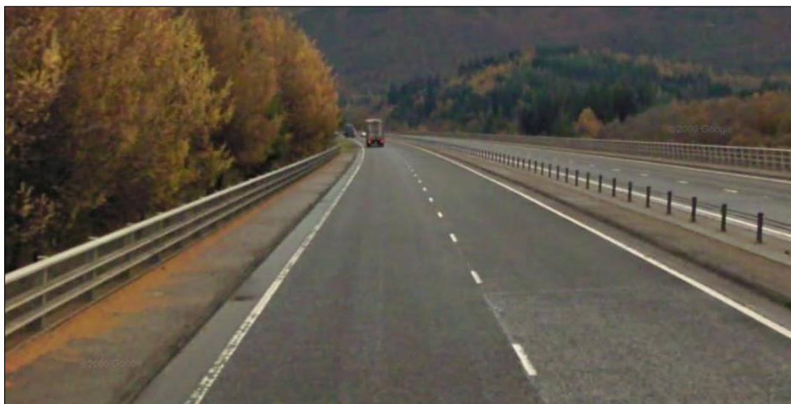
Figure 4.15.31.A – A9 600 Killiecrankie Viaduct South Bound
