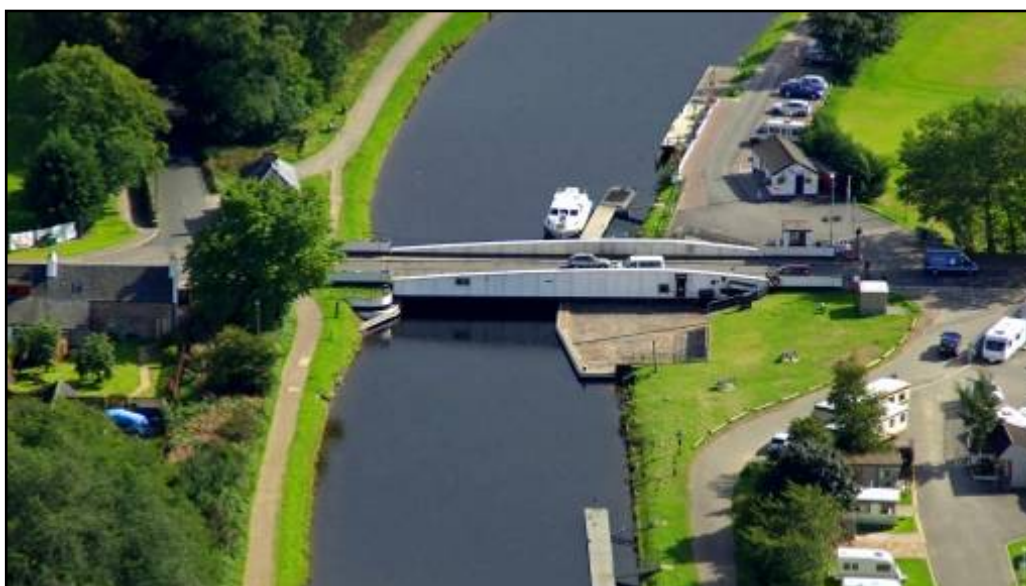
Figure 4.15.111.A – A82 1490 Tomnahurich Swing Bridge
