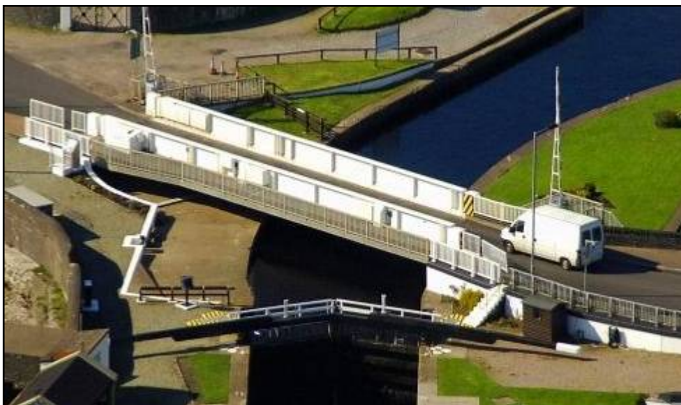
Figure 4.15.119.A – A83 240 Ardrishaig Swing Bridge
