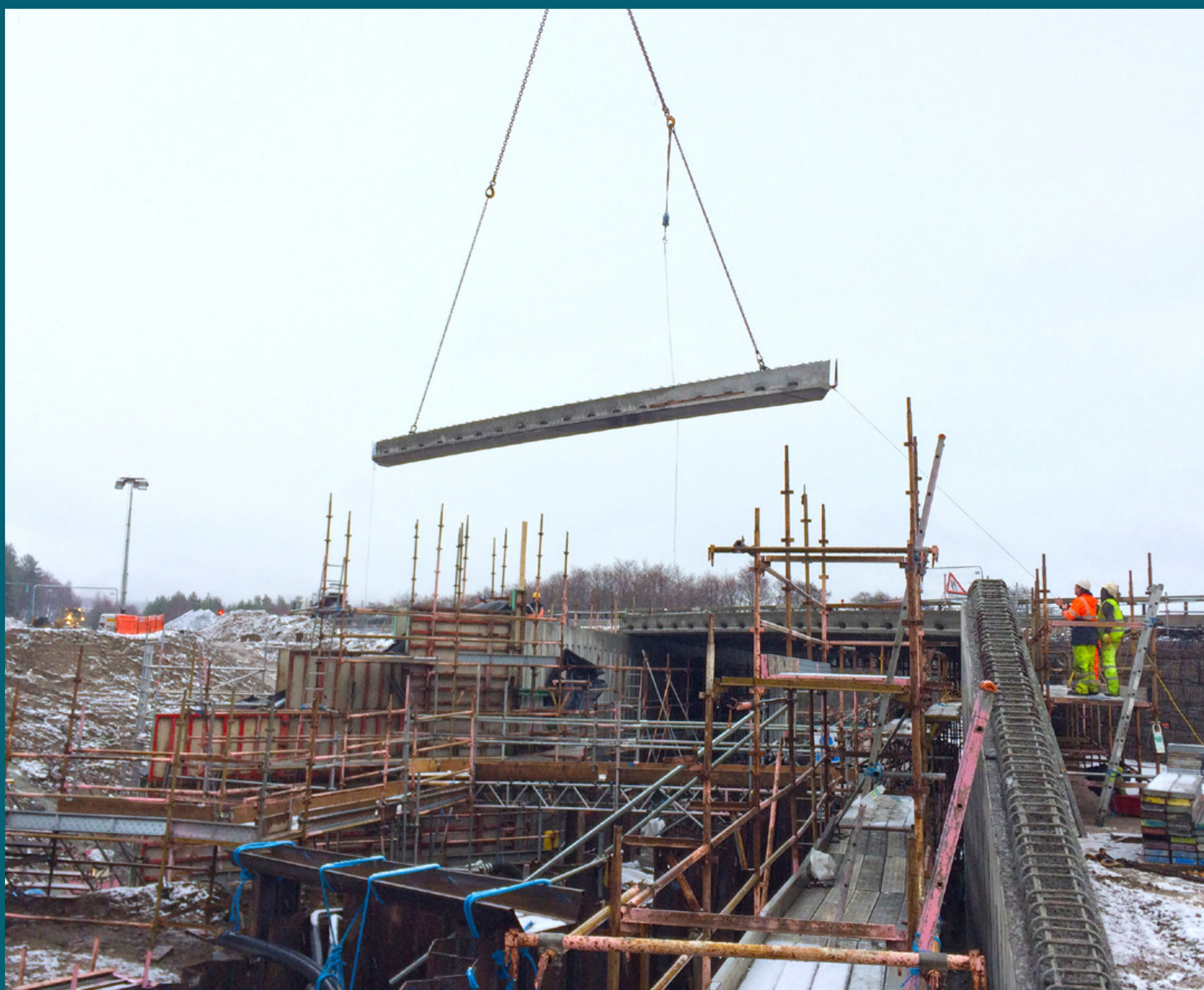
Example of Kinraig underpass under construction
