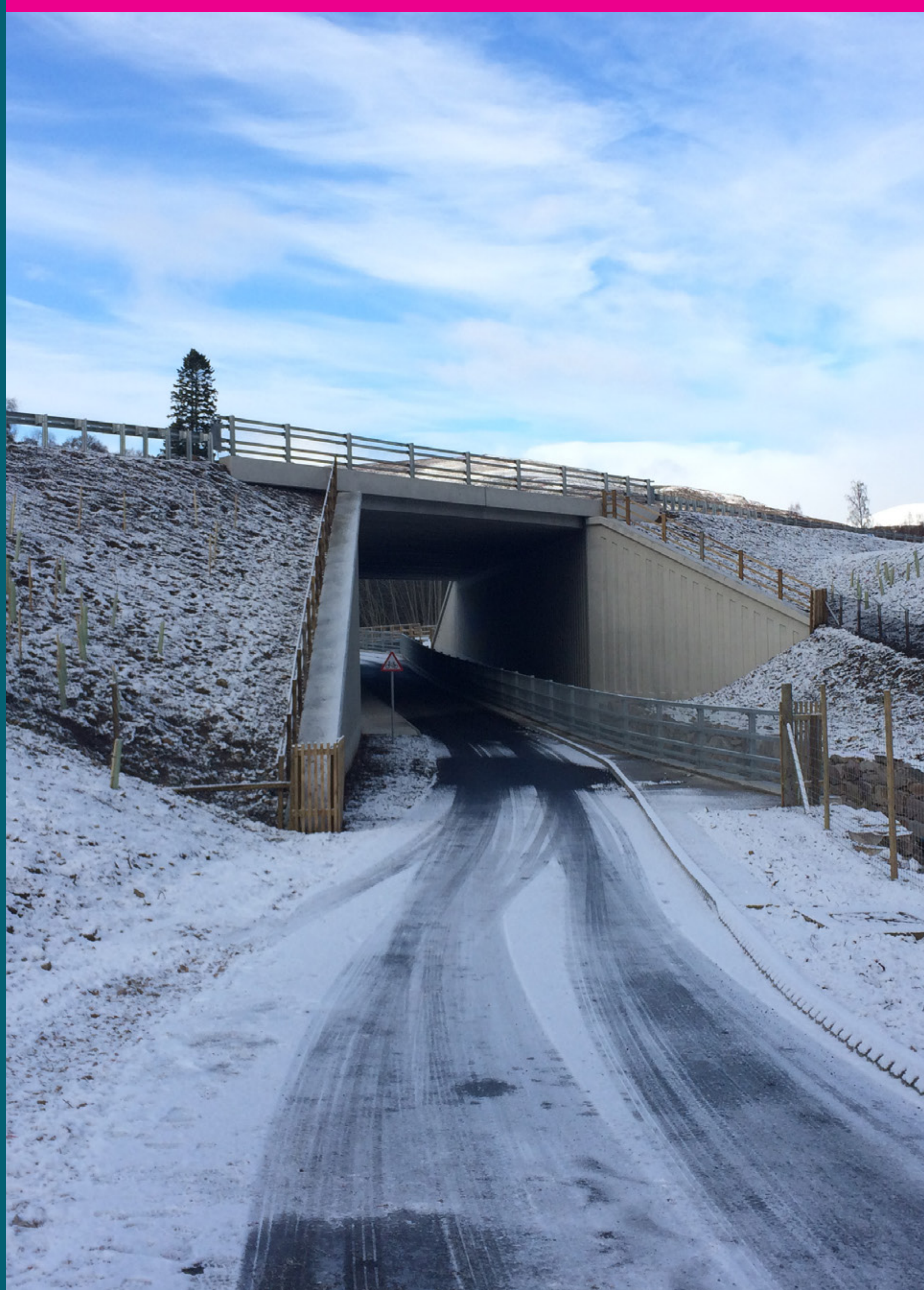
Example of Kincaig underpass (completed)
