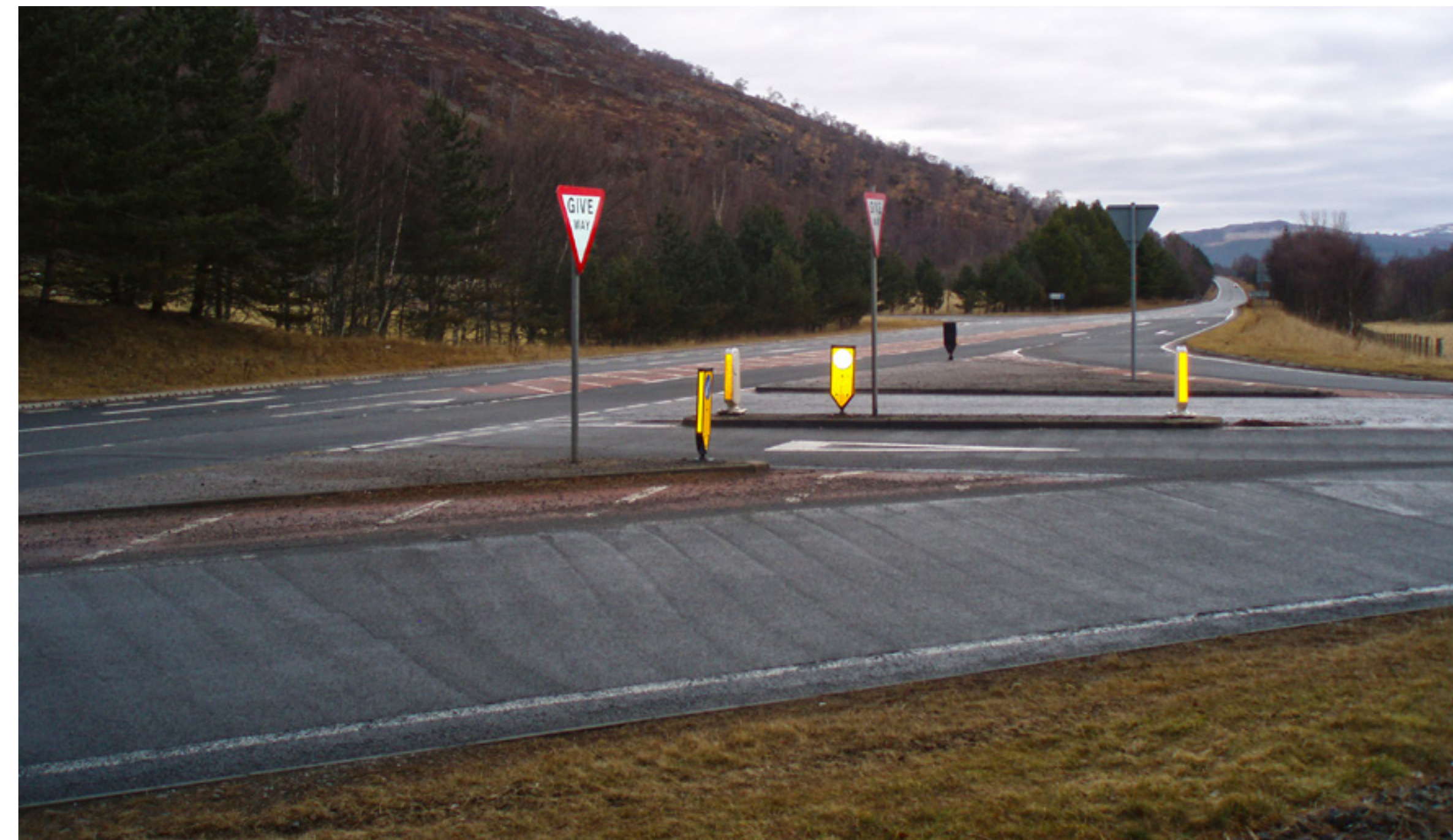
Existing Aviemore South junction
