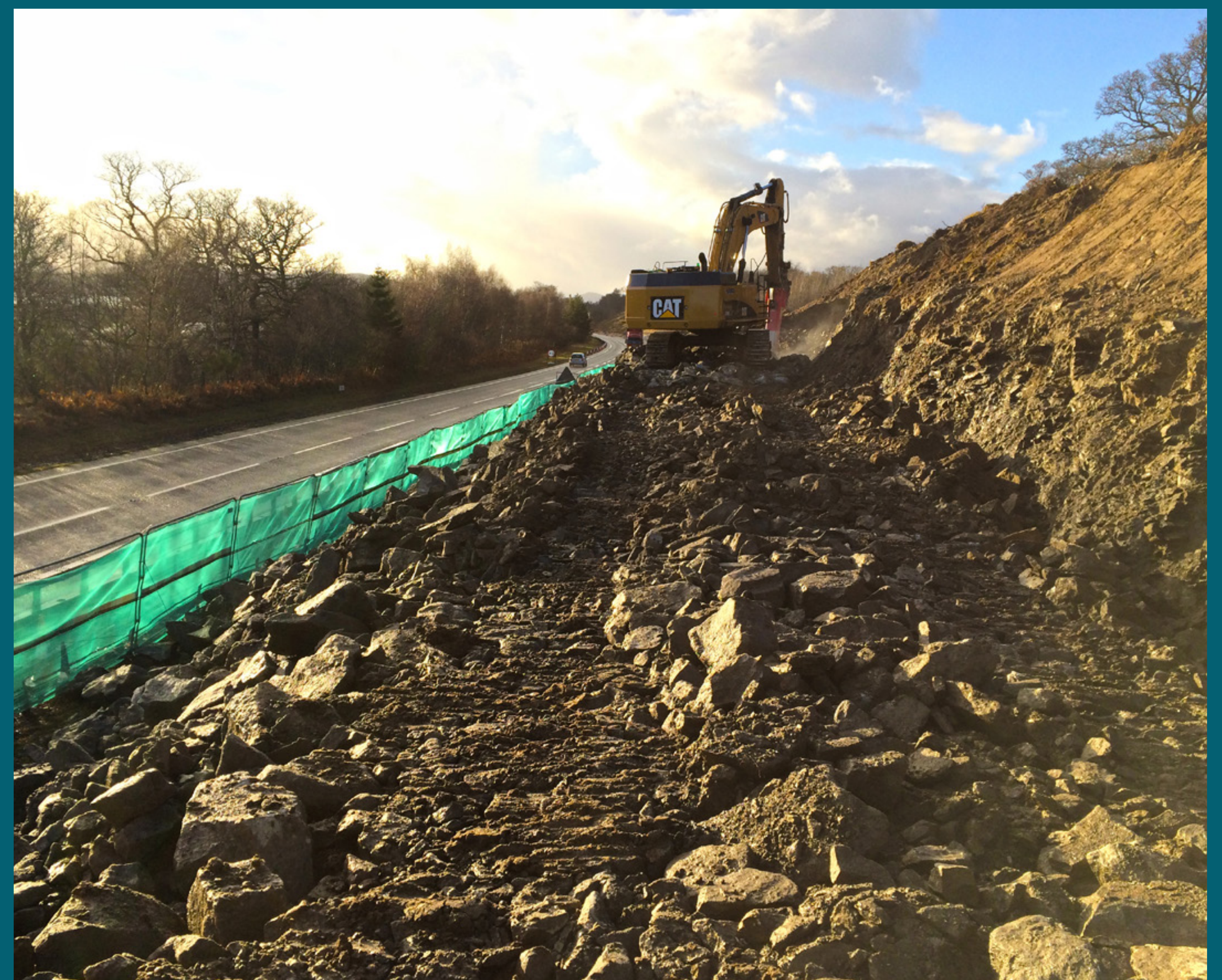
Example of Kinraig roadworks under construction
