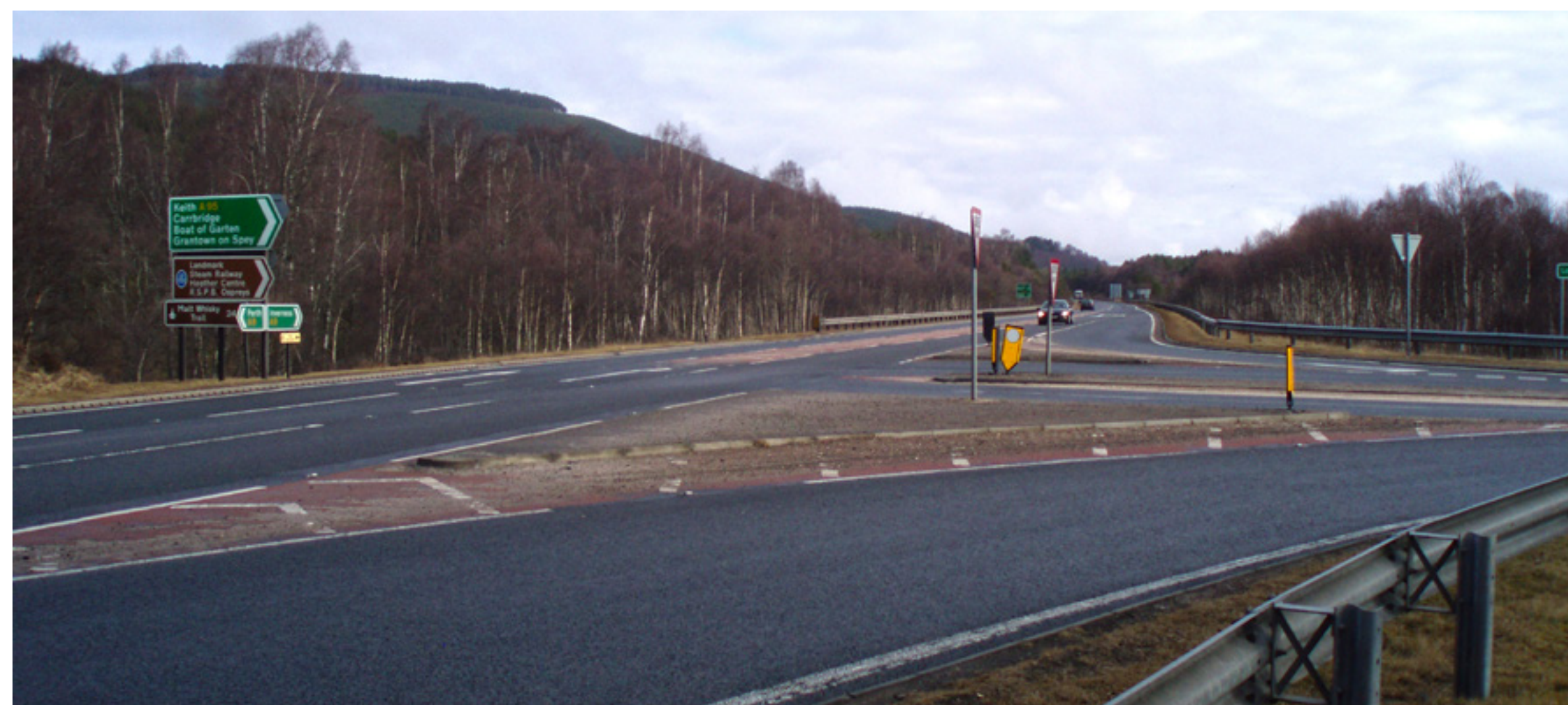
Existing Granish junction
