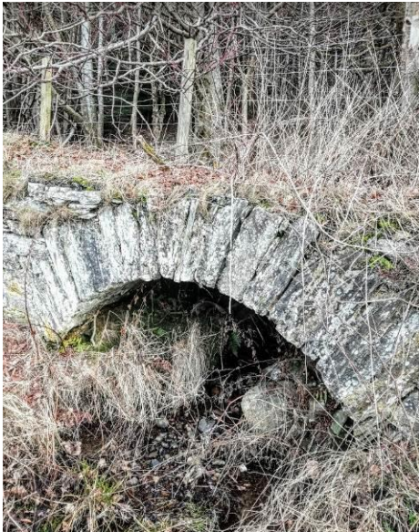
Photograph 15.23: Detail of the span of the Possible military bridge/culvert near Westhaugh of Tulliemet
