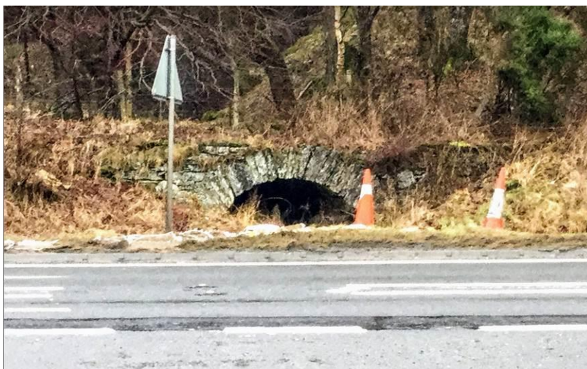
Photograph 15.22: Possible military bridge/culvert near Westhaugh of Tulliemet (Asset 781)
