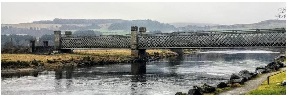
Photograph 15.17: Dalguise Railway Viaduct Over River Tay (Asset 747)
