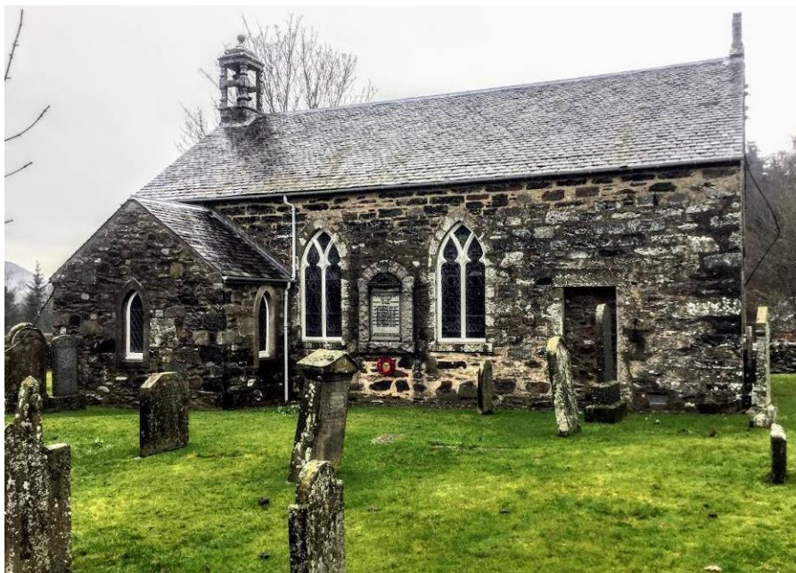
Photograph 15.10: Dowally Church (Asset 208)
