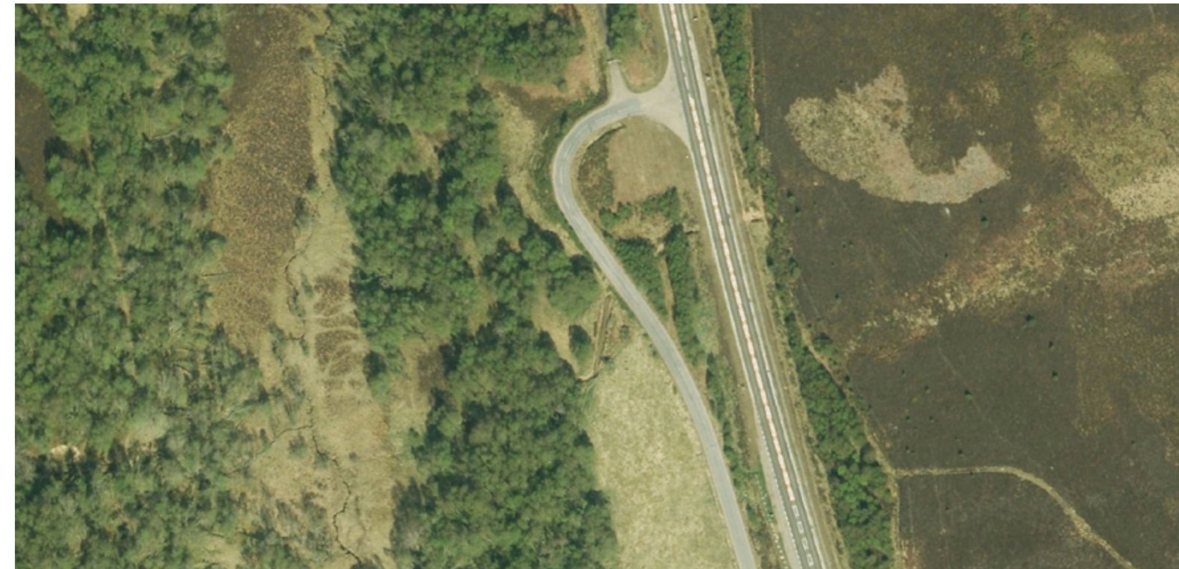
Existing Slochd junction
