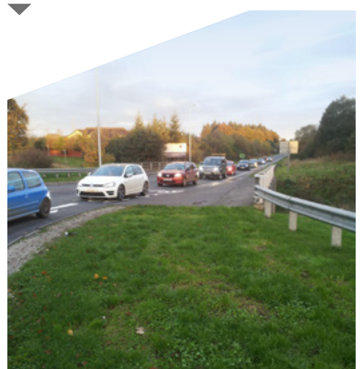
A96 Blackhall Roundabout looking west
