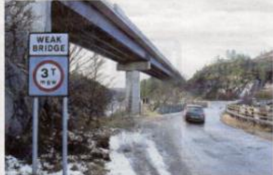
The current A9 flies over the old A9 in the foreground at Slochd
