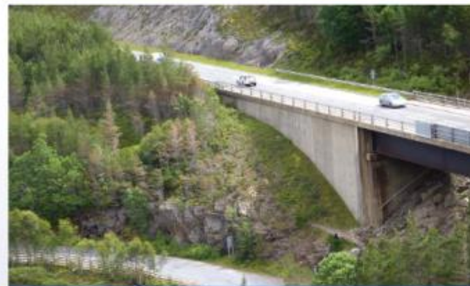
The A9 at Slochd Beag Bridge structure
