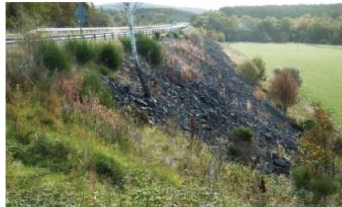
The A9 southbound at Carrbridge
