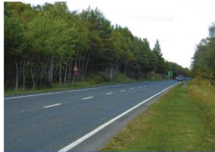
The A9 northbound on approach to Granish junction
