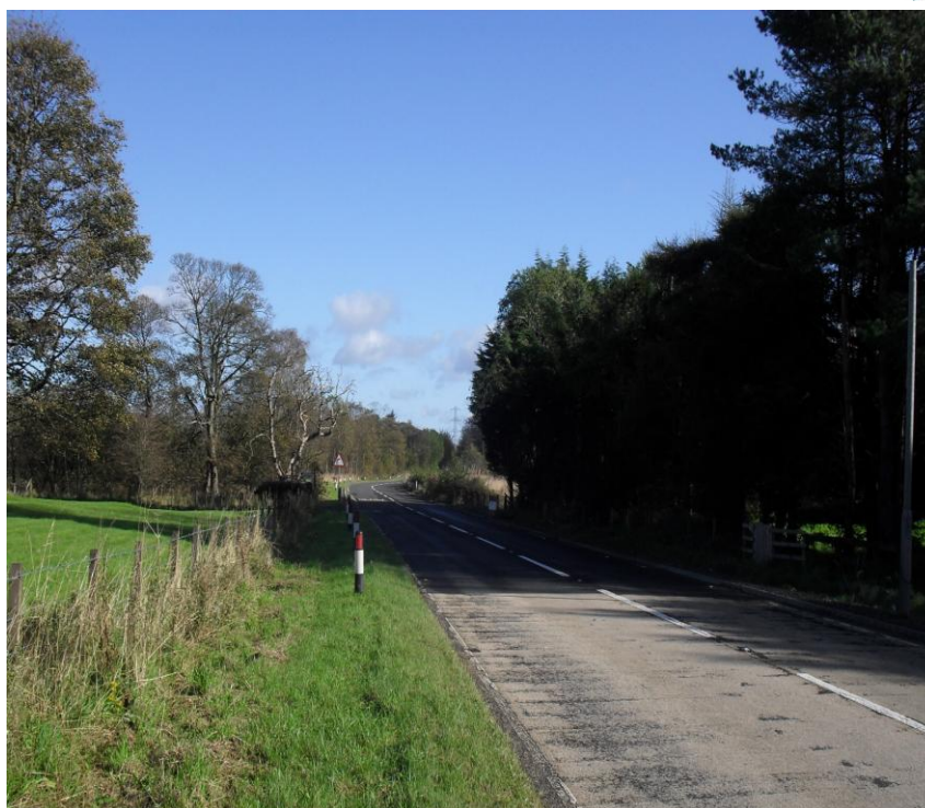
Photograph 11.5 View looking toward the northern most point of the existing road, blind right bend in the distance.
