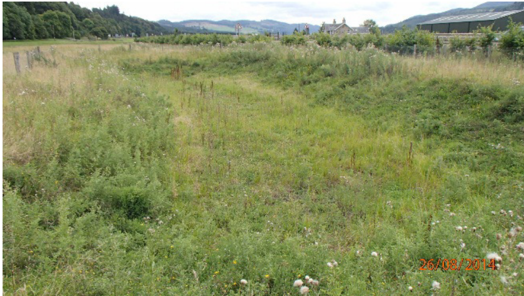
Figure 2: Dry SUDS pond with no signs of wetland vegetation
