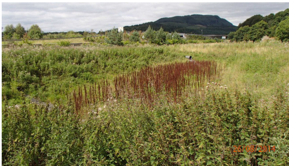
Figure 1: Dry SUDS pond dominated by dock weed
