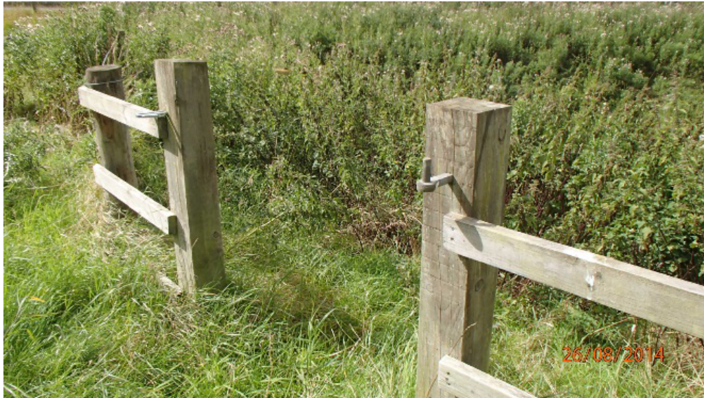
Figure 6: Missing gate at pond
