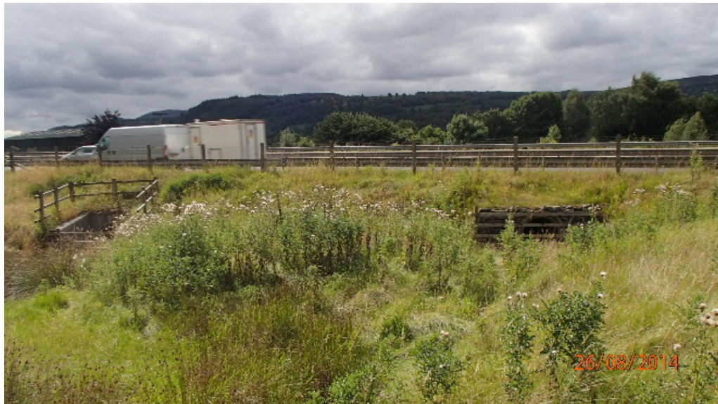
Figure 14: Mammal culvert (right hand structure) and water-crossing
