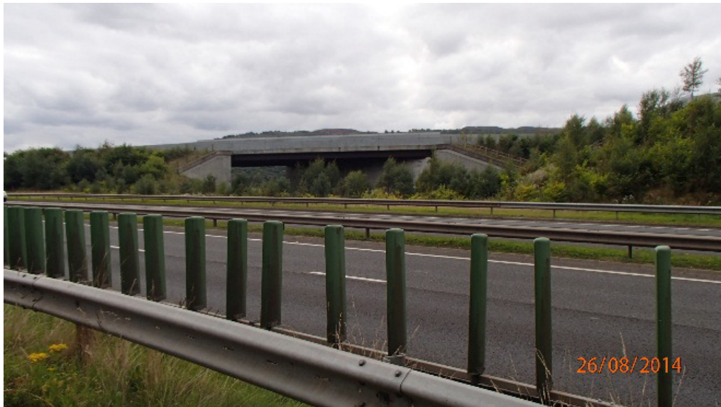
Figure 11: View of bridge over railway and planting around concrete bridge walls
