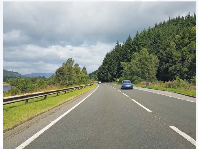
View of the existing single carriageway looking north
