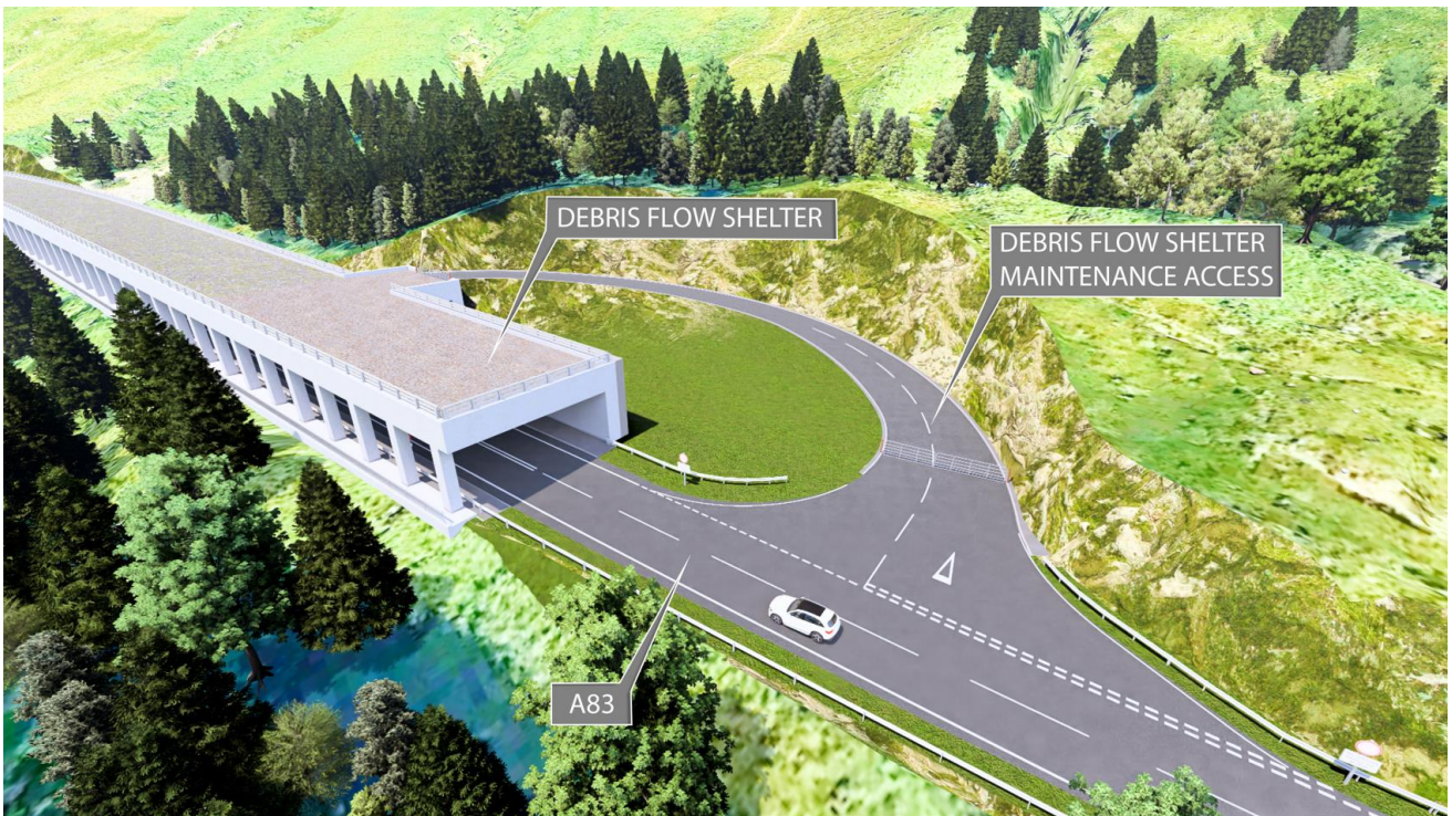
Figure 5-4 - Debris Flow Shelter – Design Visualisation
