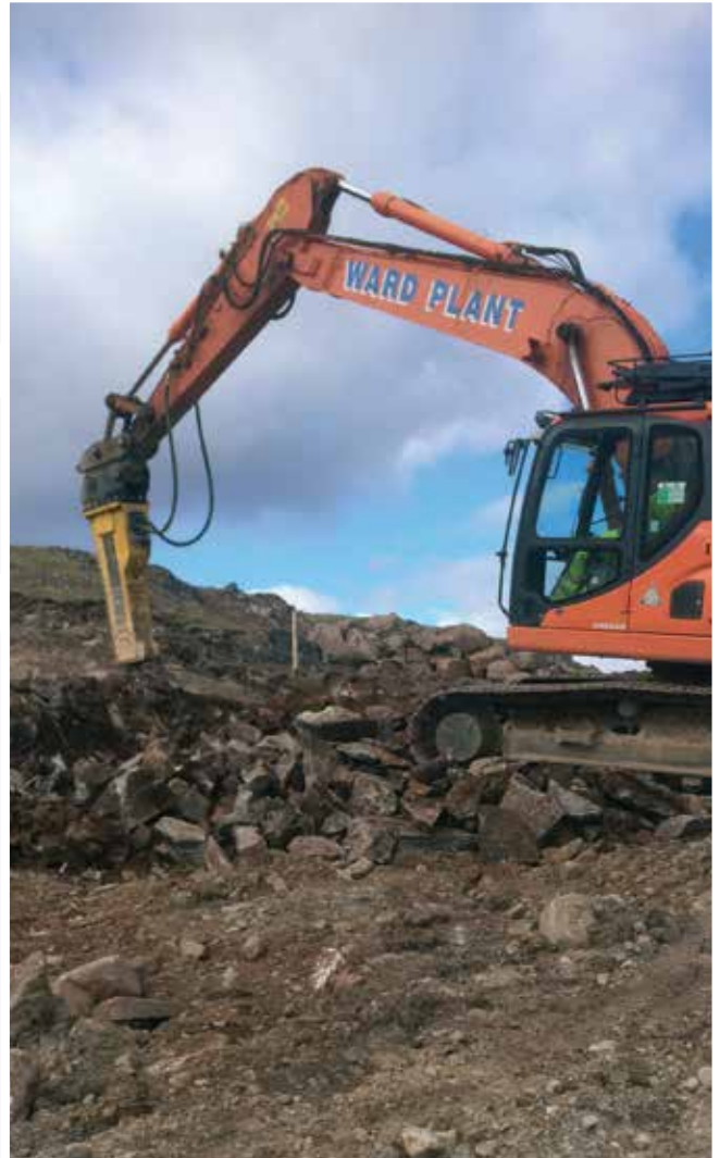
Rock-breaking at Meadowside.
