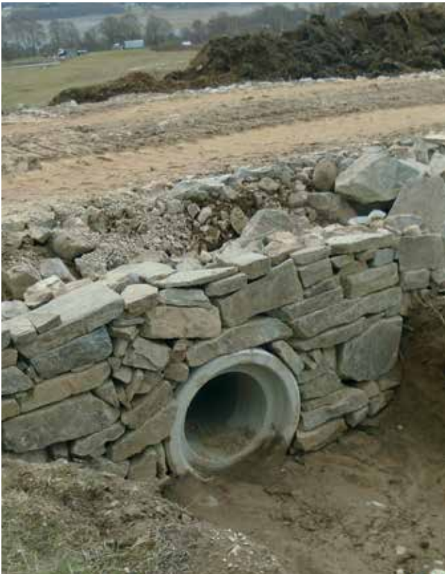
Installation of drainage on the first access route on Dunachton Estate.
