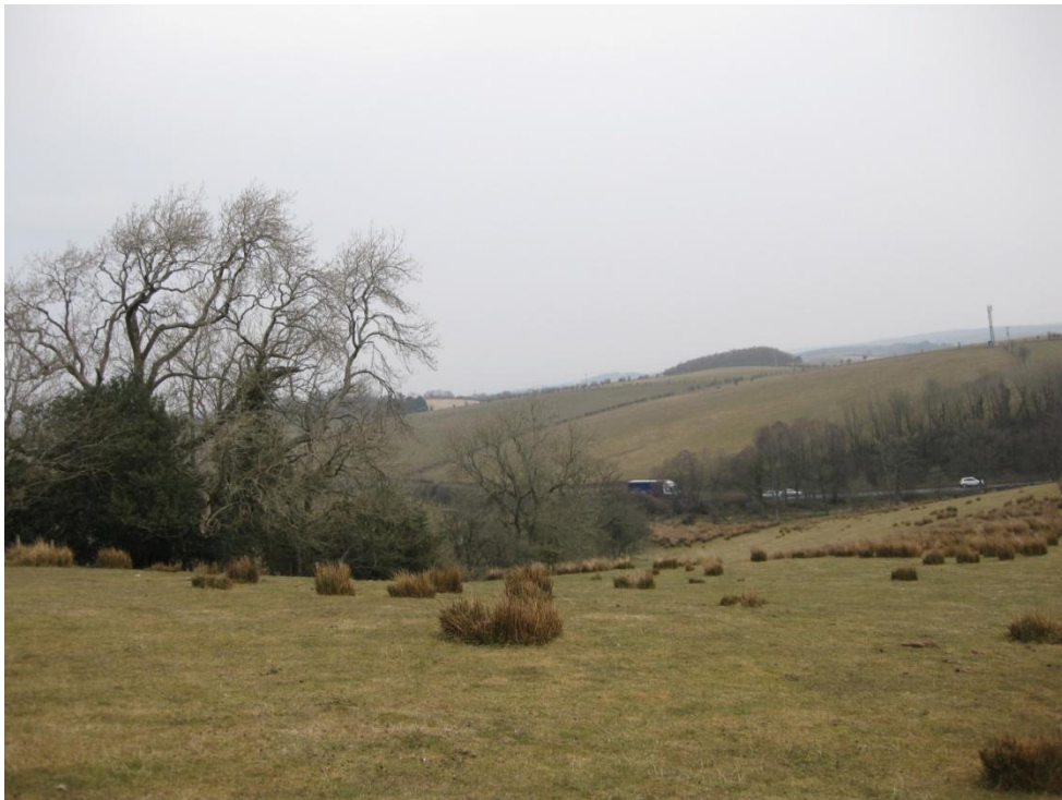
Figure 7.22 View of traffic heading north on A77 on approach to Smithston railway bridge
