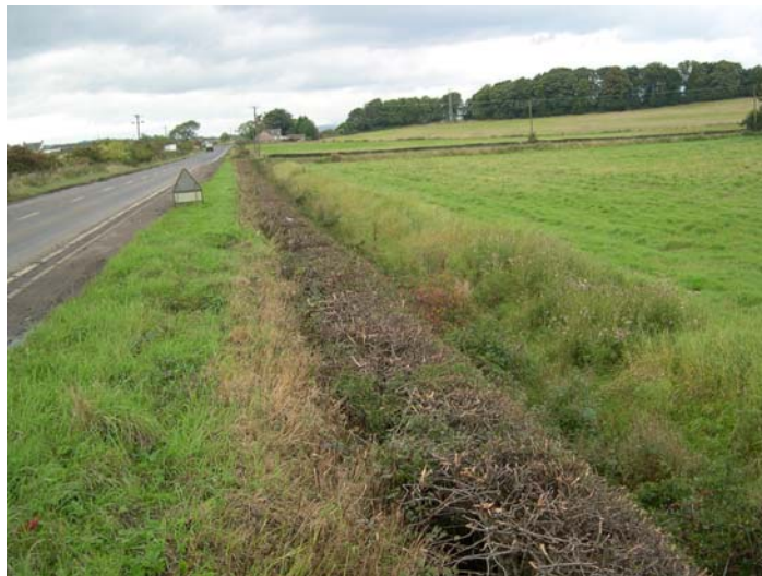
Photo. 9.7 Severely cut hedgerow at Site C (2006)
