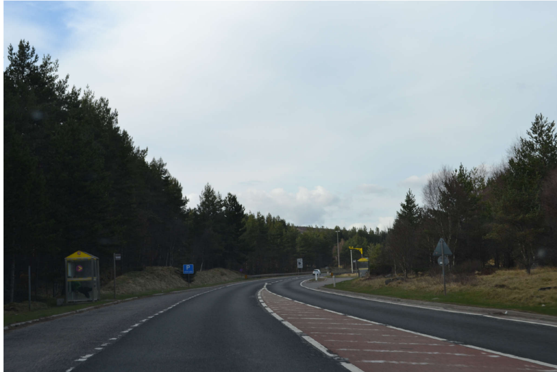
NB-01 View from north of existing Tomatin junction
