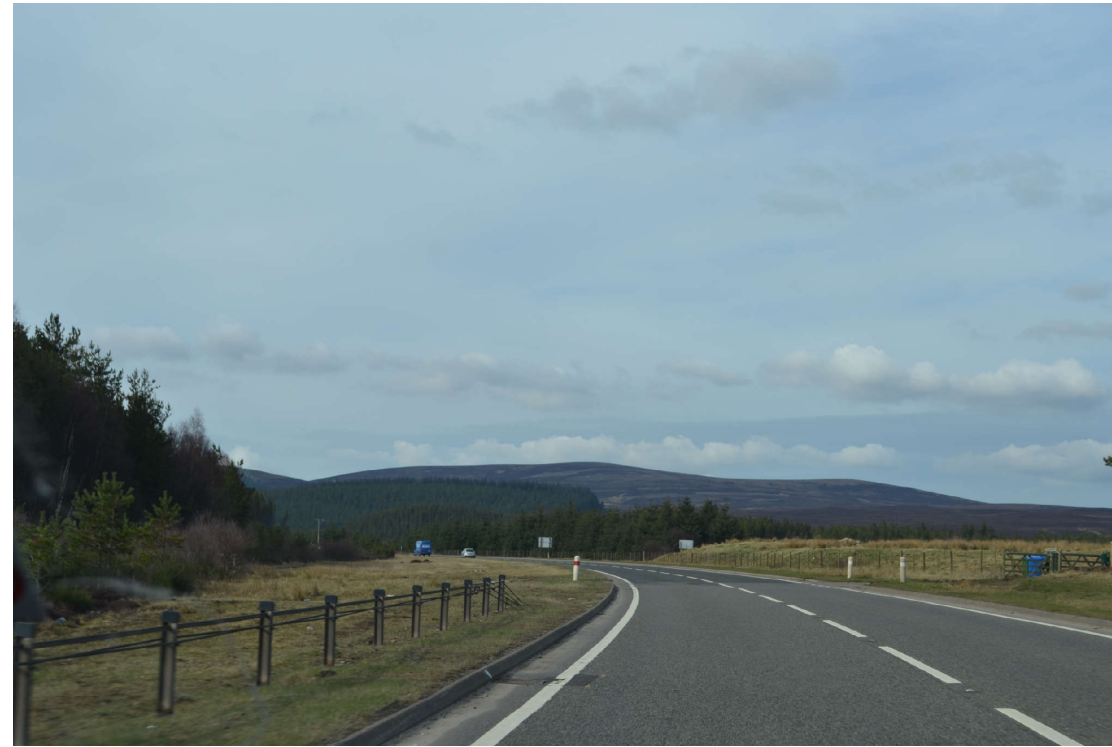
NB-02 Approaching Dalmagarry Quarry
